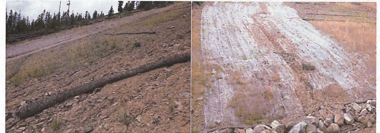
[Left]: August 7 storm damage in upper removal area. Displaced wattles and initiation of rills (looking southwest). [Right]: Initiation of gully erosion at the base of the erosion control blanket (looking northwest).
