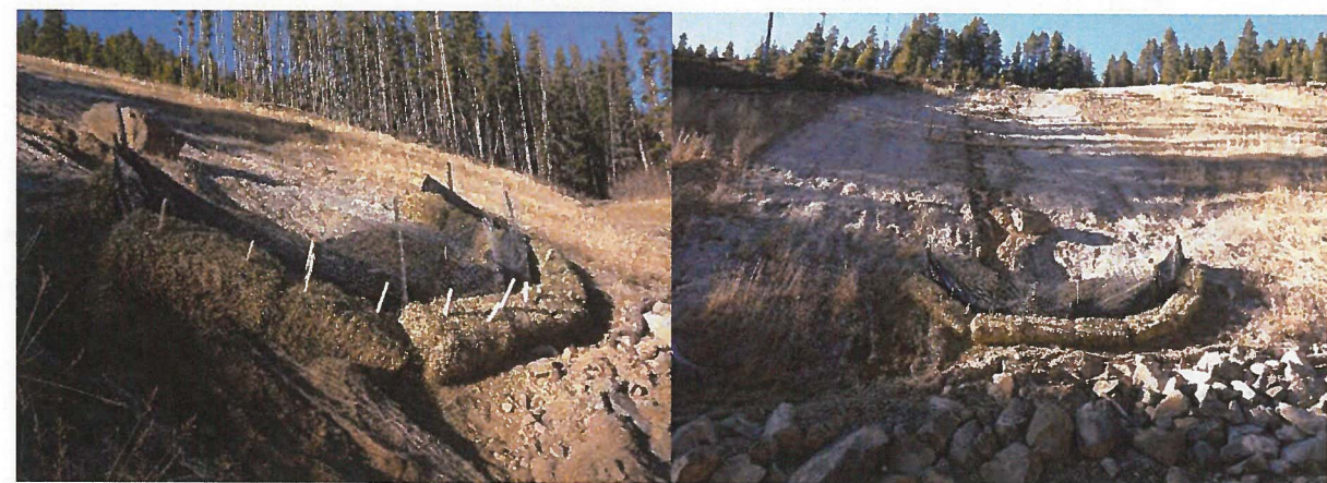
[Left]: Reinforced silt fencing used to prevent sediment from reaching No Name Creek. Silt fencing was anchored by trench excavation, steel fence posts, and straw bales secured with wooden posts (looking northeast). [Right] Silt fence below with additional erosion control wattles above to slow down water and sediment movement into the gully. Riprap at the bottom of photo is just above the No Name Creek Channel (looking west-northwest).
