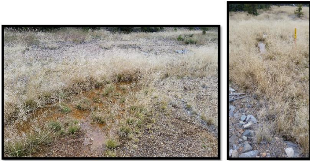
Figure 3: (Left) Sih-mem Creek adit water infiltration area above a residential yard, (Right) a partially collapsed culvert under Carpenter Road.
