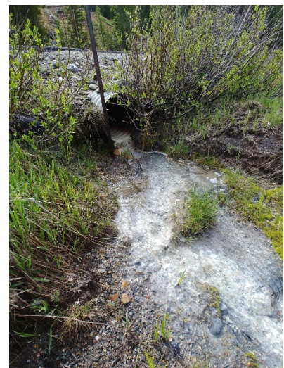
Figure 11. Mineralized outflows exiting the culvert below Montezuma Rd entering downstream wetlands. Photo taken 6/17/19.
