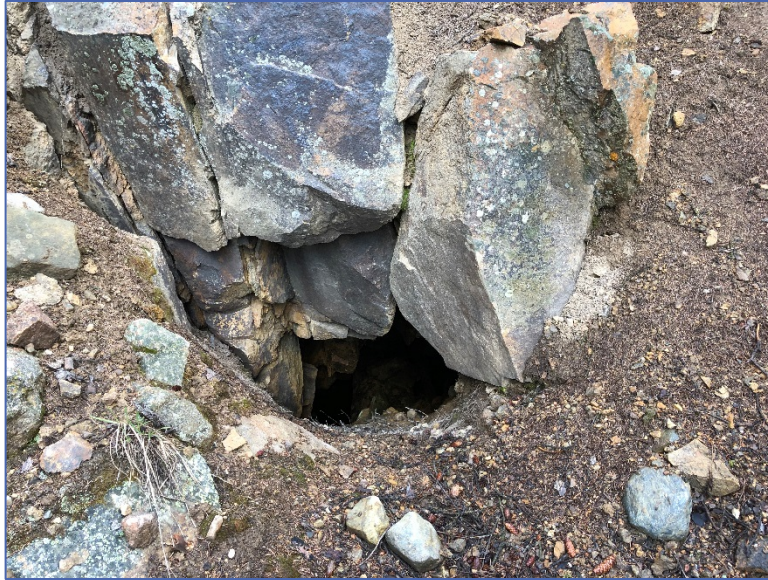
Figure 12. Flooded opening above the Manila Lode site in line with the seep location. Workings are flooded, and timbers are visible within this opening. The entrance of this feature is approximately 3 feet by 4 feet. Photo taken 6/17/19.
