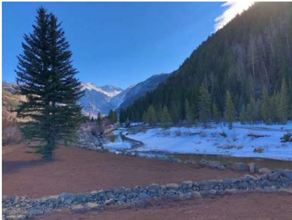
Completed North Riverbank Lining and Arm
