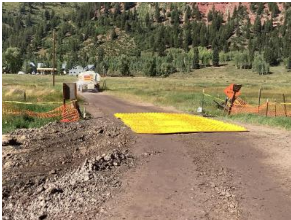
Contractor installed construction mats to help ensure all debris is removed from dump truck tires prior to leaving the site. Additionally, a water truck sprays down the road to minimize dust.
