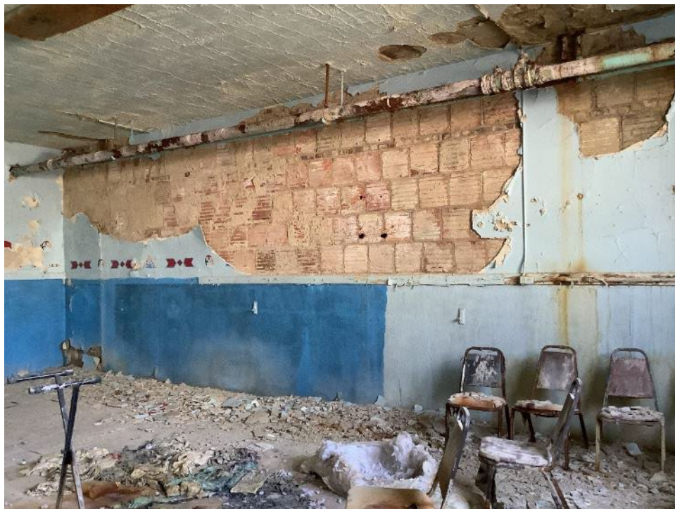
Interior of former St. Katherine school building. Showcasing deteriorating conditions of shared wall with adjacent Pacelli Building. Date: 03-09-2022
