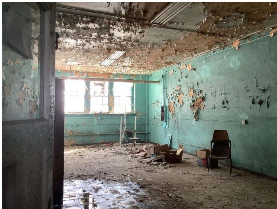
Interior of former St. Katherine school building. Deteriorating conditions exposing asbestos containing material and lead based paint. Date: 03-09-2022
