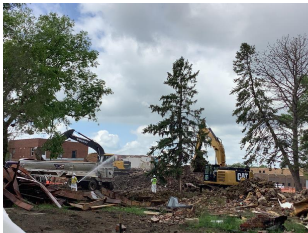
Loading debris into haul truck with dust control
