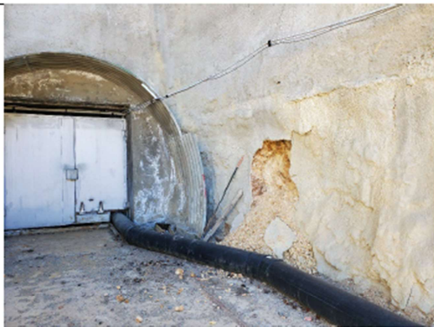
GK Photograph 3: Image of the shotcrete on the walls of the portal.
