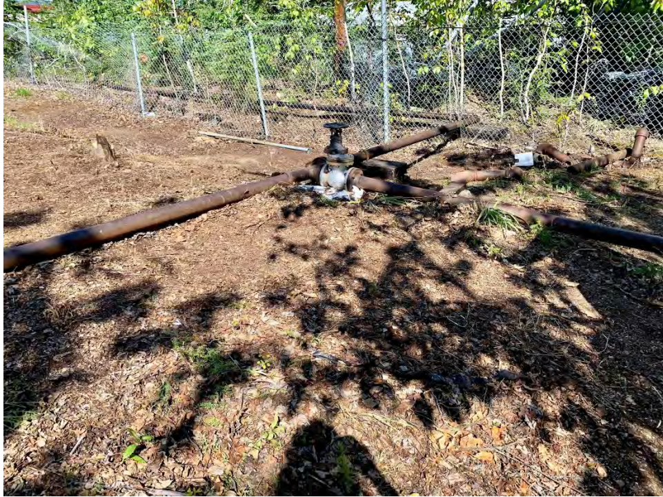
Photo 1- Northeast facing view of the three-way valve. July 14, 2020.
