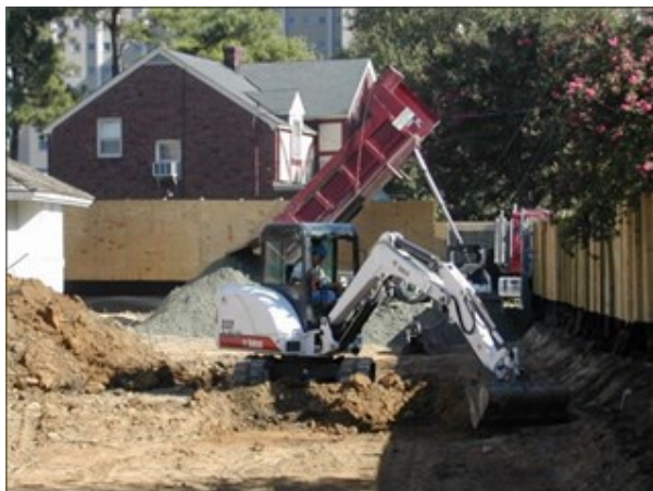
Figure 2. Excavation of a yard with lead contamination
