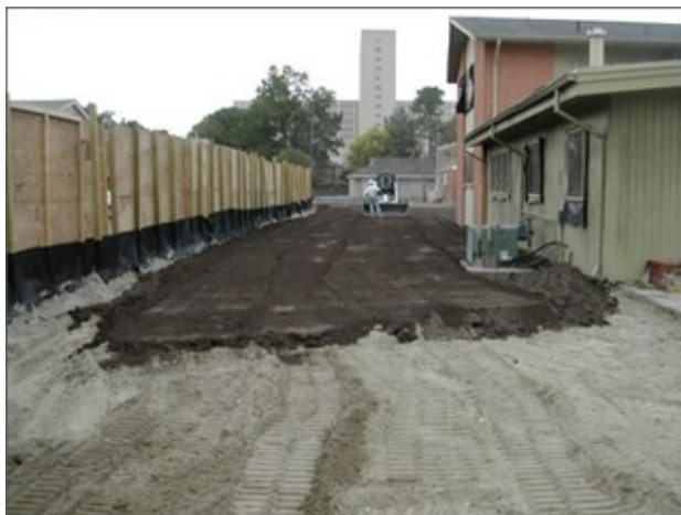
Figure 3. Backfilling an excavated yard with clean
