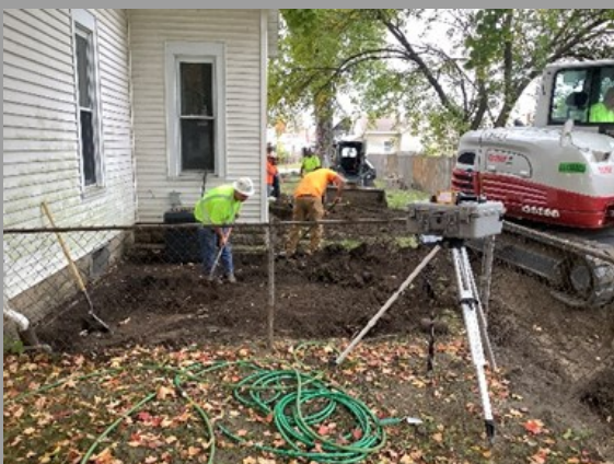
Figure 6: Air monitoring device to detect air-
