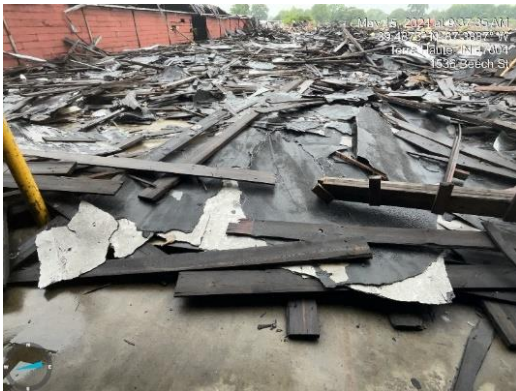
Asbestos-containing roofing material.
