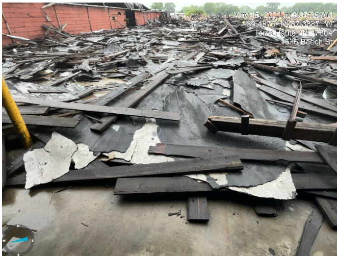
Asbestos-containing roofing material.
